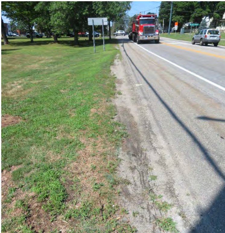
Figure 3.19 Along the edge of Route 202, scouring, compaction and lack of a curb are visible. (LG HL 9Aug2019 (254))
