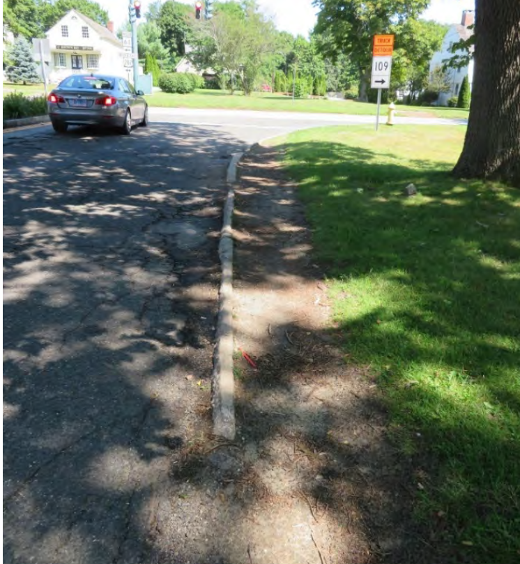
Figure 3.18 A segment of broken and missing concrete curb on South Street. (LG HL 9Aug2019 (221))
