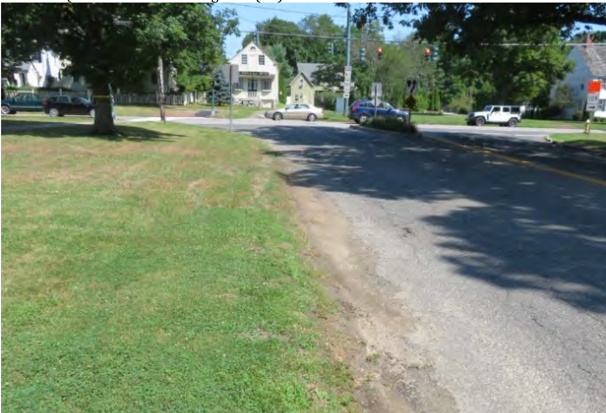
Figure 3.17 A section of streets around the Litchfield Green lack a curb and exhibit a deteriorated edge. (LG HL 9Aug2019 (218))
